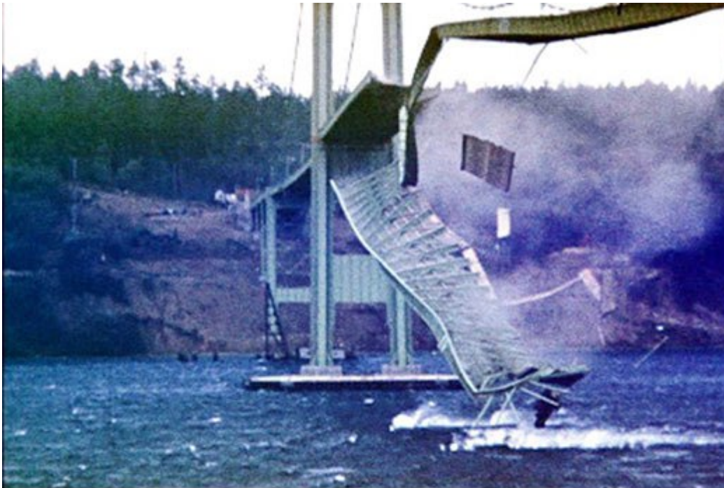
Tacoma Narrows Bridge Collapse, in color, taken from 16MM Kodachrome motion picture film by Barney Elliott.
