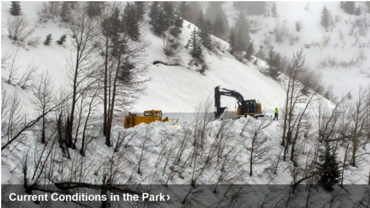
Crews are active working to reopen the Going-to-the-Sun Road
