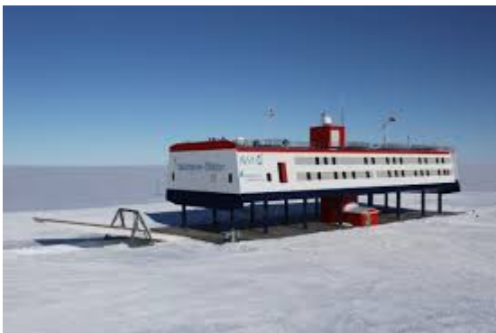
Neumayer III Station
