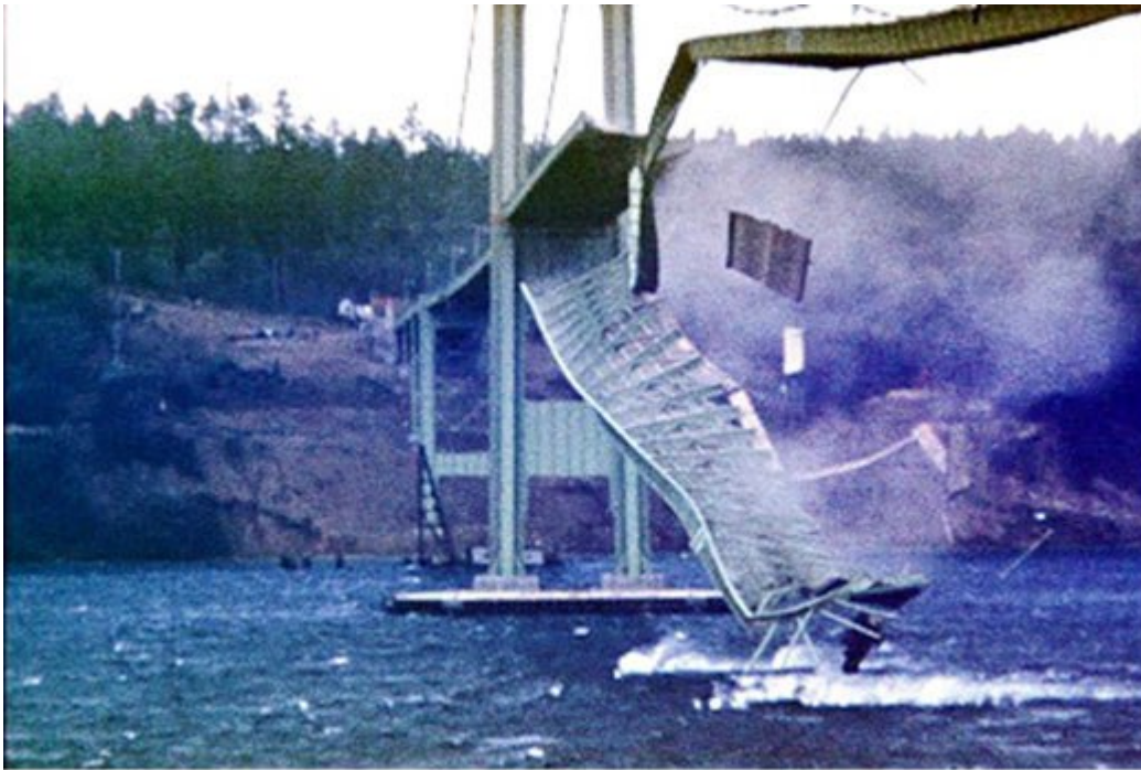
Tacoma Narrows Bridge Collapse, in color, taken from 16MM Kodachrome motion picture film by Barney Elliott.
