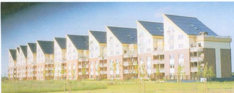
Fig. 2-29: Multifamily house with solar roof in Rostock
