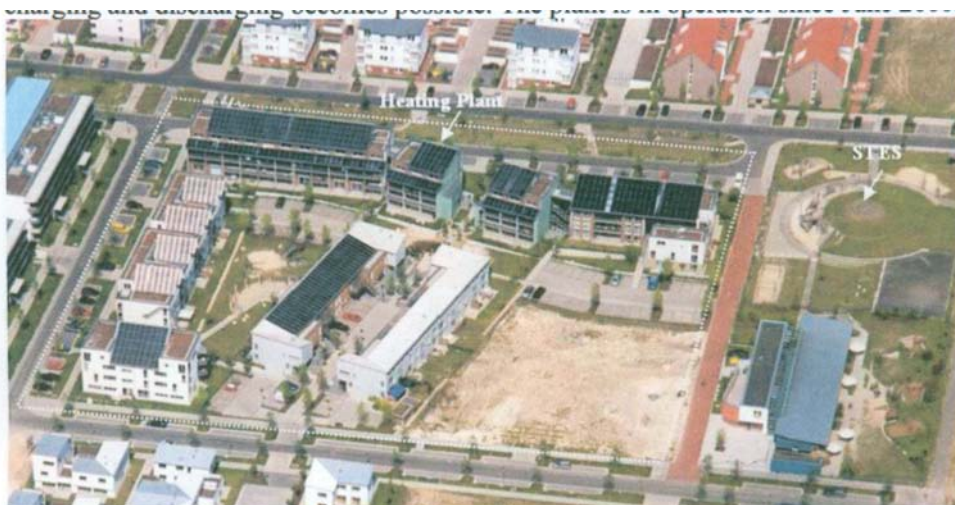
Fig. 2-30: CSHPSS in Hannover (source: Gockell)
